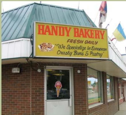
Handy Bakery before new façade
